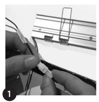
Cut 12-13mm (0.47-0.51") wide slot to required length. Bring through power feed and make connection to GROOVE In.
